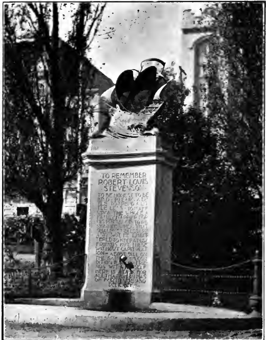
STEVENSON MONUMENT, PORTSMOUTH SQUARE
